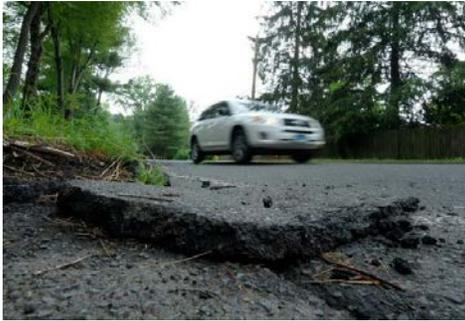
A hilly, winding road in New Fairfield, Conn., is cracked and recessed on the edges. Almost half the state's major roads are rated 'poor.' / Robert Deutsch, /USA Today
