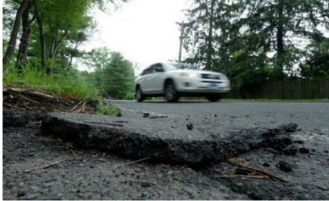
**A hilly, winding road in New Fairfield, Conn., is cracked and recessed on the edges. Almost half the state's major roads are rated 'poor.' / Robert Deutsch, /USA Today**
