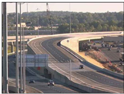
Two new flyover bridges opened early Saturday morning at the interchange of i-85 and Highway 316.
